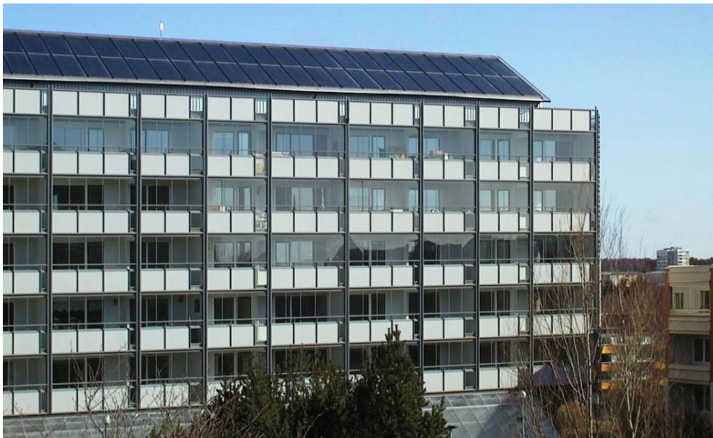
Roof module collectors on a renovated multifamily building in Gårdsten, Göteborg.
