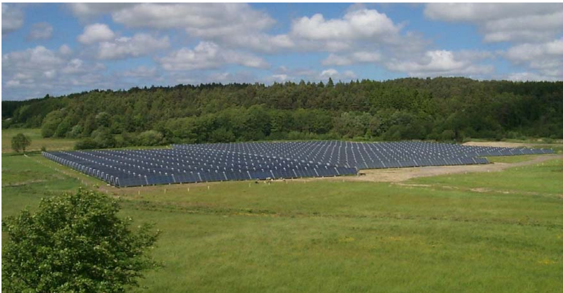
Solar district heating plant with 10 000 m 2 large-module collectors in Kungälv, Sweden.
