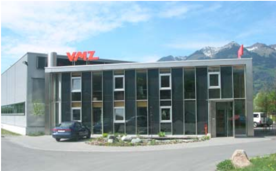
Fig. 3: Facade integrated collector at a commercial building (Source: DOMA)
