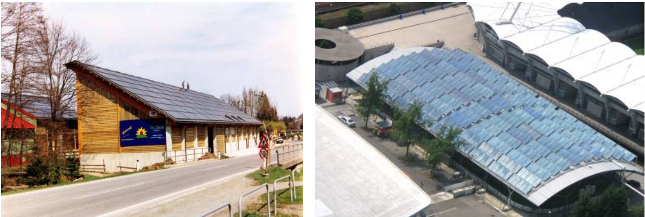
Fig. 9: Left picture: Solar assisted biomass district heating plant, Eibiswald with an installed capacity of 875 kW th , (1250 m 2 collector array). Right picture: District heating plant in Graz with an installed capacity of 980 kW th , (1400 m 2 collector array). Source: S.O.L.I.D.
