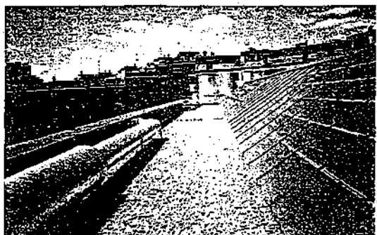
The 53 kilowatt system of the library includes four rows of skylights consisting of opaque and semitransparent modules.
